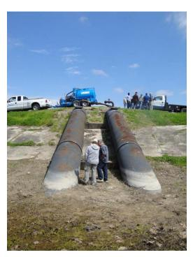
Triton Vacuums can rapidly evacuate air out of a vessel or pipeline and create the reduced atmospheric pressure that allows the siphon to form and gravity to take over the flow...in this case, to the opposite side of the levee.
