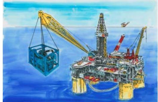
One decommissioning project consisted of flushing and removing about 10,000 feet of 2" and 2 1/2" lines, all below the waterline. The lines were in lengths ranging from 1800 to 3000 feet each. The deepest section was about 17' at pipeline crossings. Vacuuming with a "Triton 500" unit was continued until the line was flushed at 1-1/2 times the line volume, at which point decommissioning work could continue.
